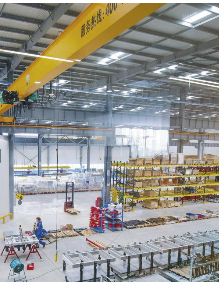
Around 8,000 m 2 of additional production space in the newly opened factory
